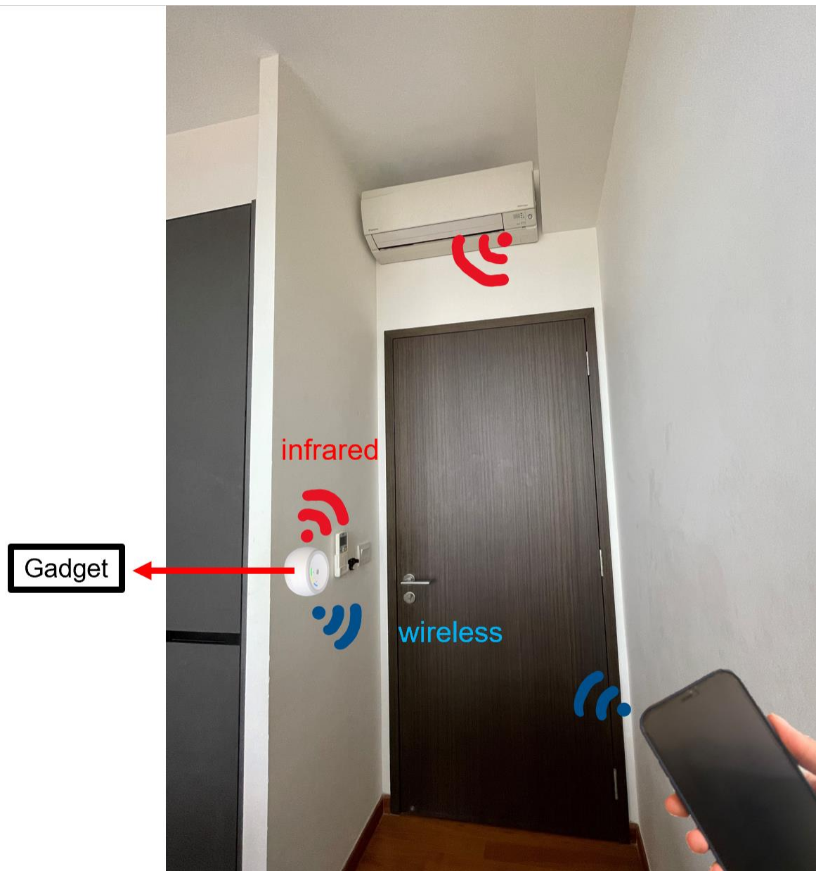
Figure 3.1: How the gadget connects the app to the air-conditioning
